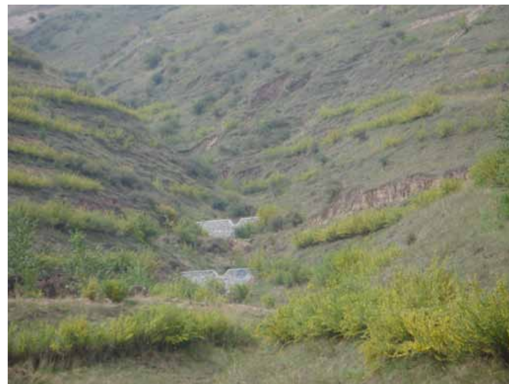
Figure 2: Series of sediment control dams (Photo credit: World Bank Office Beijing)
