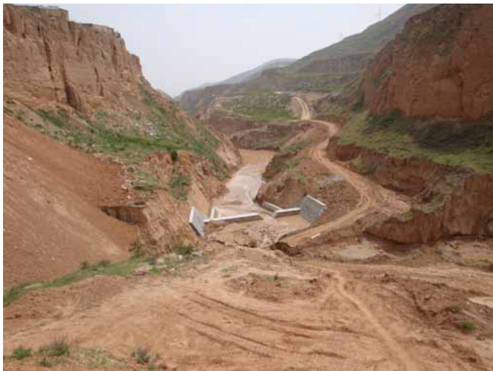
Figure 1: Warping Dam in Gansu province, China. (Photo credit: WorldBank office Beijing)
